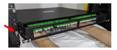
**4.1.2.3** Install additional screw on the mount bracket then tighten all the screws to secure the panel in place.
