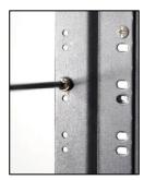
**4.2.2.2** Place the panel mounting brackets over the screws allowing the panel to rest on the screws.
