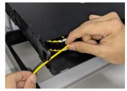
**4.1.3.2** Do the same process for the remaining Jumper cables, then after all MPO Jumper cable are routed put the Rear Cover back on the chassis.
