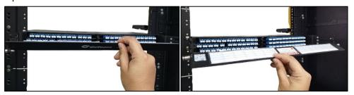
**4.1.4.2** Spread out other adapters to isolate the desired adapters from the others, then remove the dust caps.
