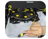
Take the outer-end of MPO jumper and pay-out the cable up the desired length
